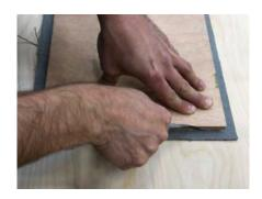
Make sure that the perimeter is well fixed to the base and cut the covering following the edge of the panel using a sharp cutter.
